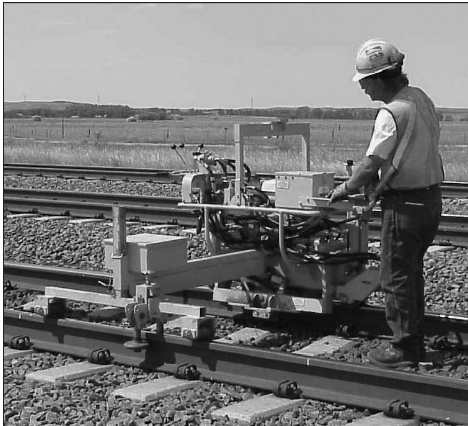
Ultra Clipper applies/retracts up to 3 different styles of resilient fasteners
