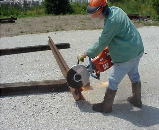
Top Rail Cutting
