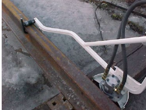
Web Grinder on the rail.
